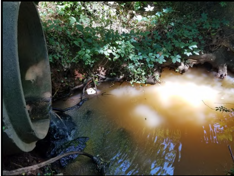
9 NWW-2A. Culvert just east I-77. No upstream aquatic passage due to position of culvert above streambed.
