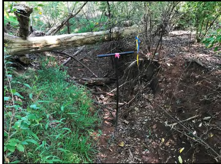
2 NWW-1. Between culvert and property boundary. Eroding banks typical of areas around slopes. Channel is also incised.
